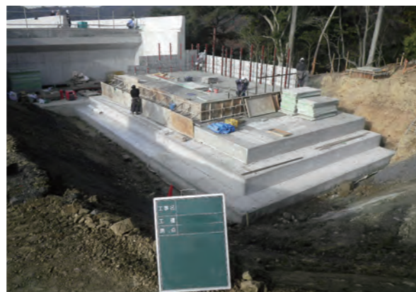
▲型枠組立解体状況
